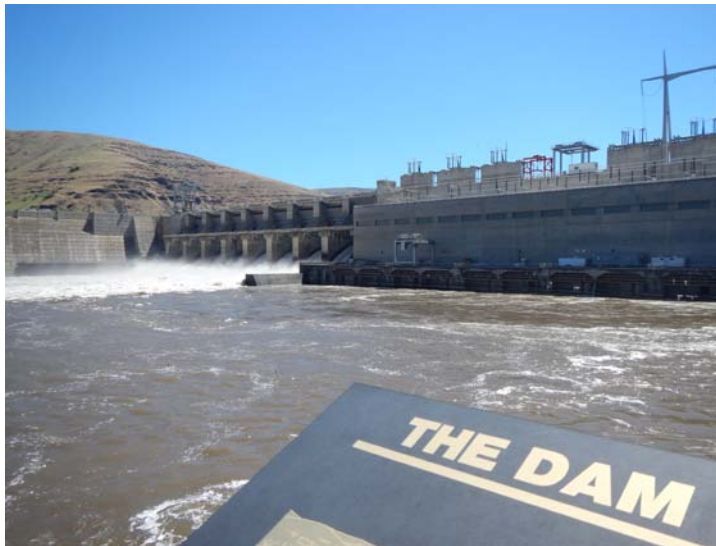
Lower Grante Dam, Snake River Brett Haverstick FOC file photo
